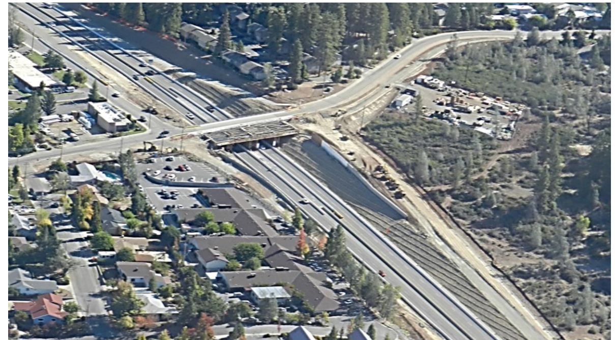
Dorsey Drive Interchange construction site with exit and entrance ramps and bridge widening under construction
