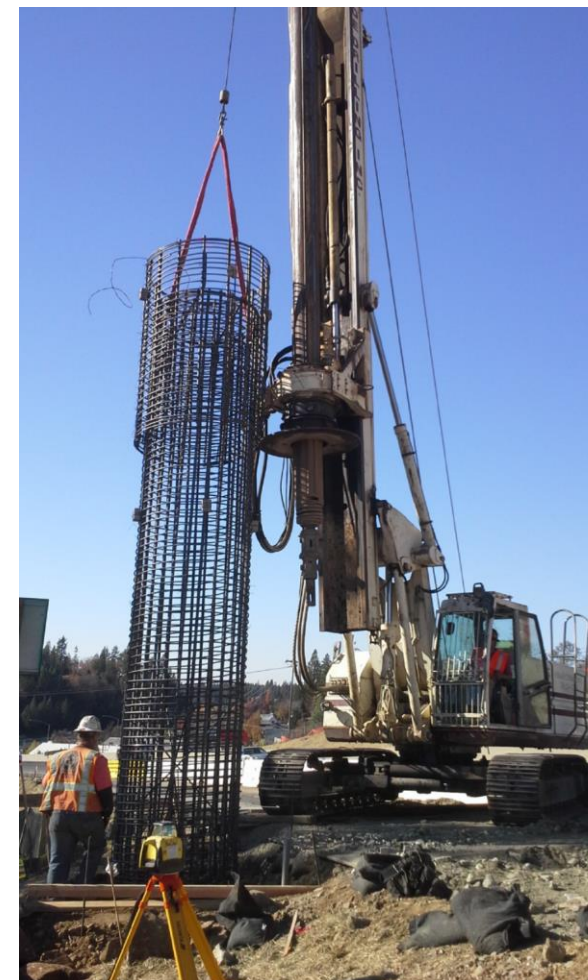
Drilling hole 50 feet deep to install pile for freeway sign
